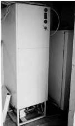
The system could be controlled so that it delivers heat to the space-heating loop independently of any space heating needs if there is a risk of overheating in the system.
