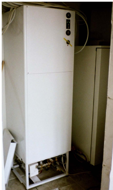
Figure 2: Storage tank and other components integrated in cabinet
